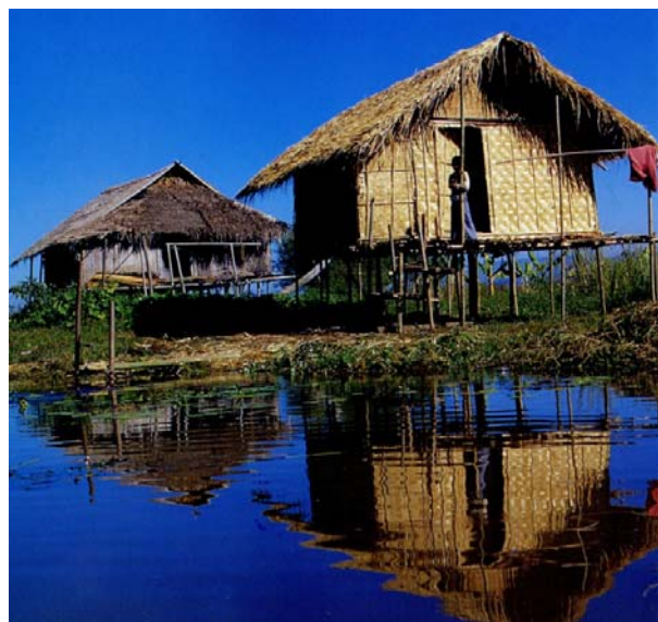
Figure 5.1 Bamboo and palm house on stilts, Inle lake, Burma. (Vellinga et al. 2007)
