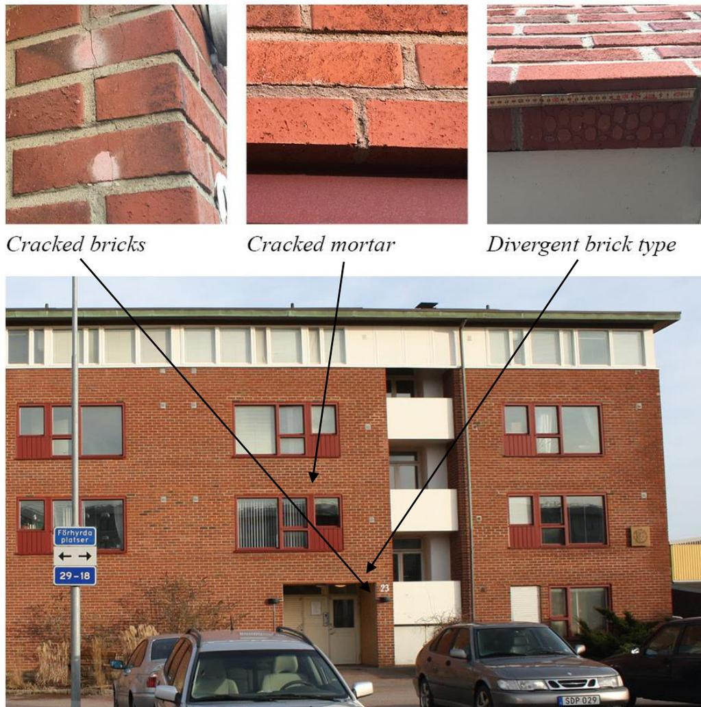
*Figure 3.4* Some damages and deviations observed during the visual inspection. More pictures are available in appendices.
