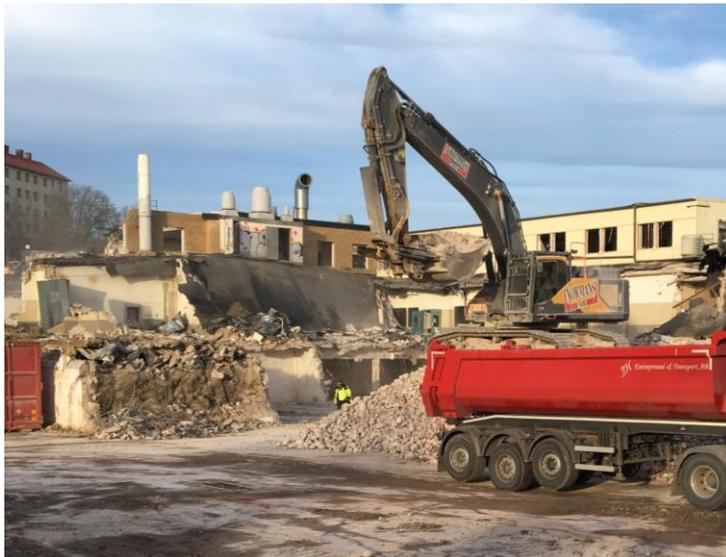
*Figure 4.6* Truck in use during the demolition of Fixfabriken in Gothenburg, March 2019. 50-75% of the bricks do not break during demolition and remain reusable.
