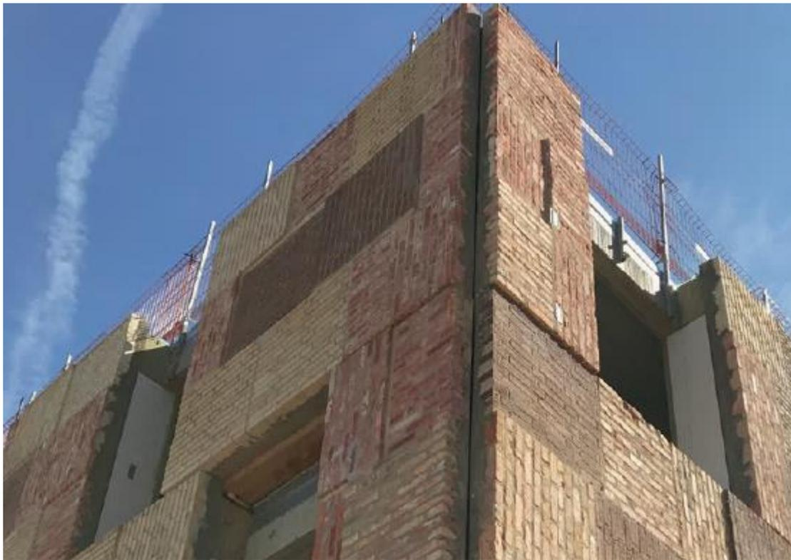
*Figure 2.8* The facade elements with brick modules during construction. Reprinted with permission from Lendager Group.
