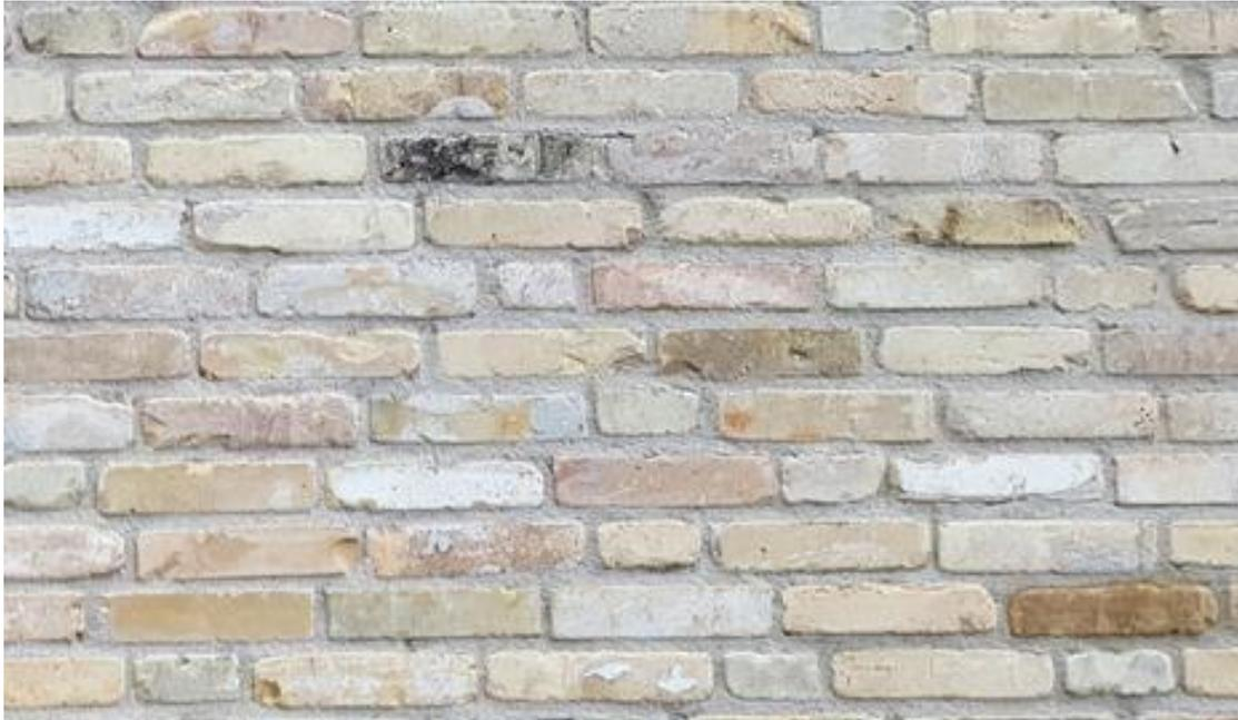
*Figure 2.2* The bricks of Furutorpsparken. The texture is relatively rough and mottled. Reprinted with permission from Brukspecialisten.
