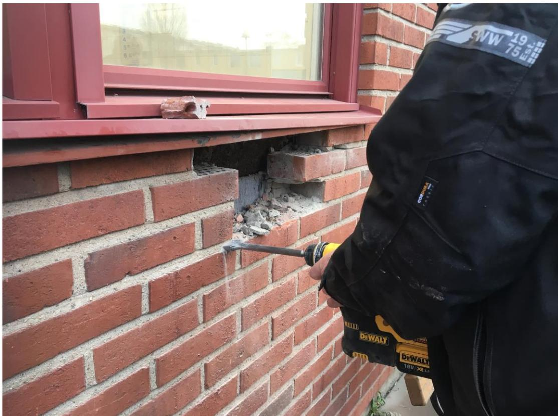
*Figure 4.2* Deconstruction of five bricks. The mortar came off the bricks very easily and it was not possible to remove two bricks connected with mortar.
