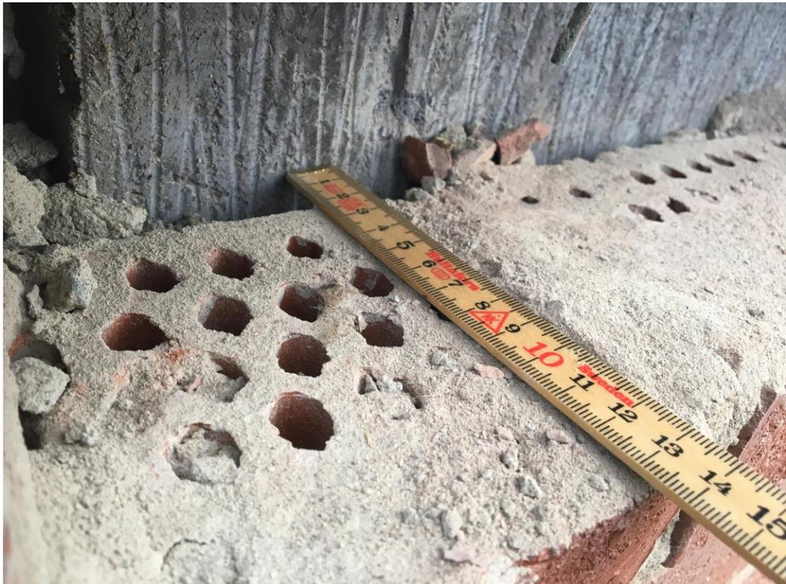
Figure 4.3 The bricks, the air gap and the lightweight concrete.
