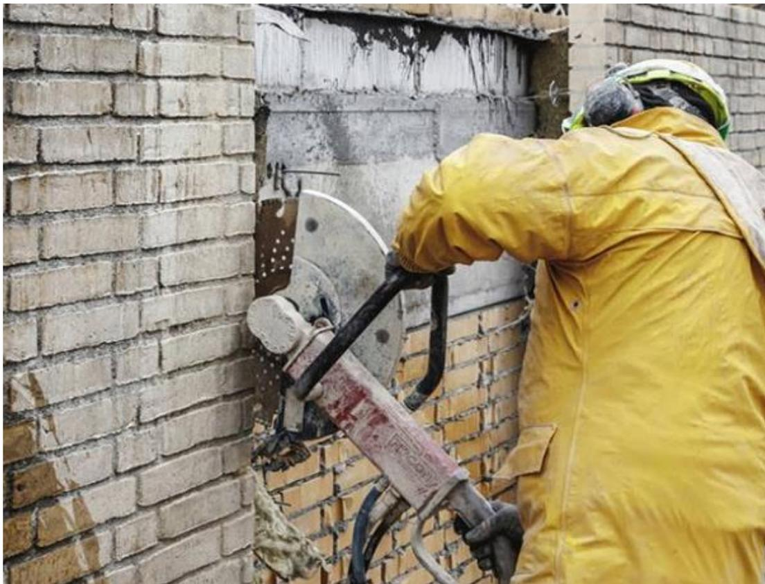
*Figure 4.7* Deconstruction of brick modules using a circular saw. Reprinted with permission from Lendager Group.
