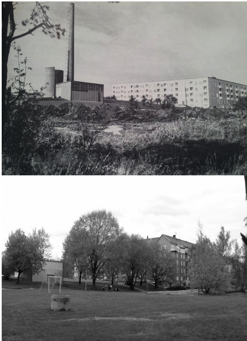
Figure 8: A view of Växelmynstgatan before and after the refurbishment. Top photo: Jan Olsson
