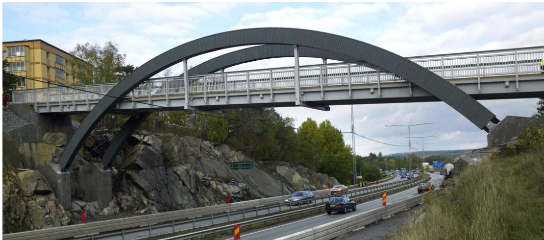
Figure 2.1 Three hinged arch bridge over E18 in Hägernäs, Moelven Töreboda AB (2010).
