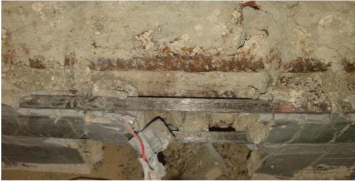
Fig : 10 Disclosour of NSM plate after cover crushing[3]
