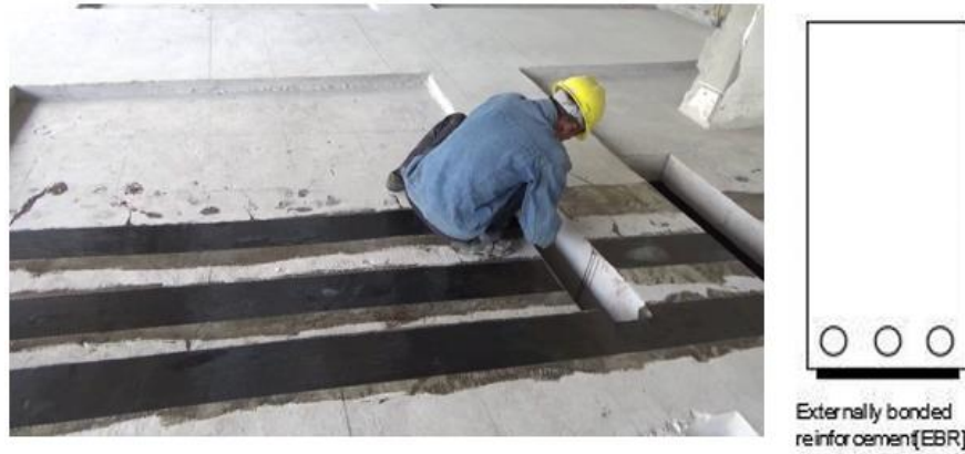
Fig:3 Application of FRP External bonded reinforcement
