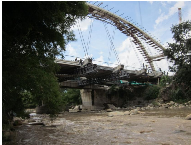
Figure 7. The construction of the new bridge over Rio de Oro
