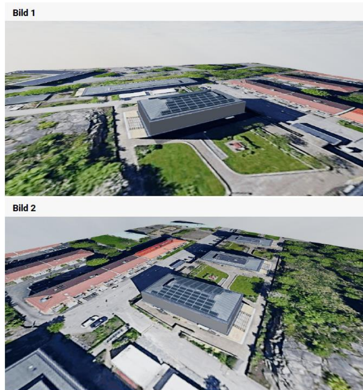
Figure 40- Replacement of solar panels on roof.
