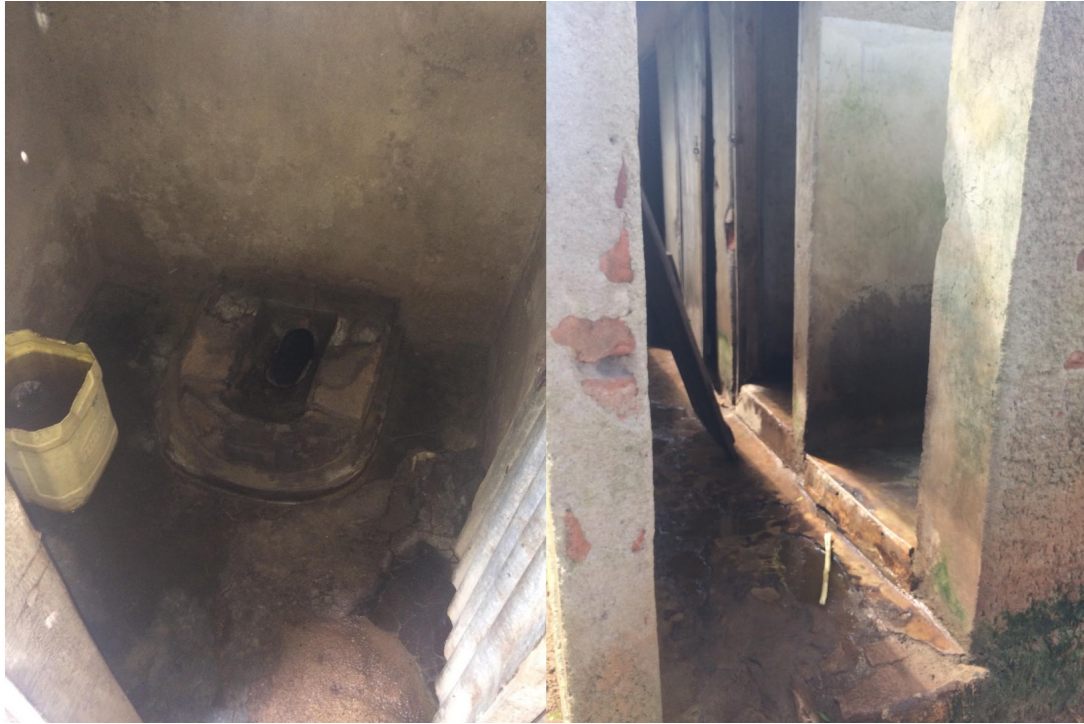
Figure 4. Left: Inside the girls' toilet with squatting commode, uneven floor and water bucket. Right: The boys' toilet stalls with uneven floors and lacking doors (Augustsson & Nylund, 2020).
