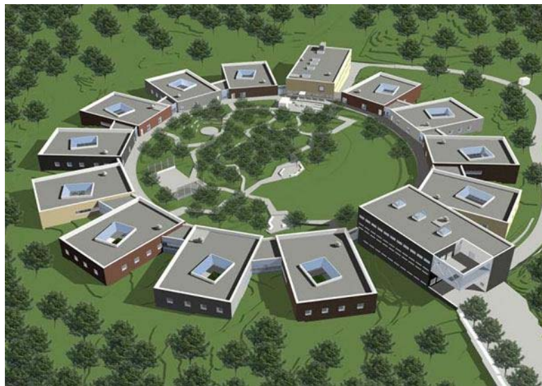
Figure 1 3D-model overview of the Brinkåsen facility.
