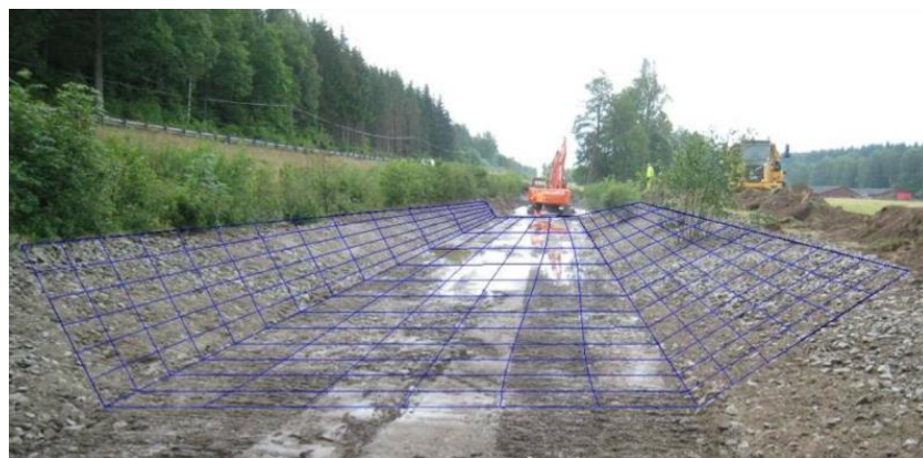
Figure 9: Illustration of model-based machine guidance. Source: Tyréns (2012).
