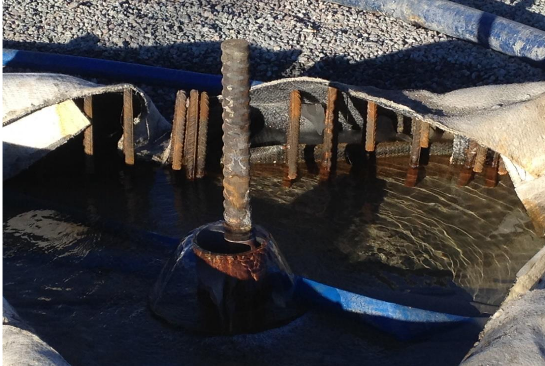
Figure 4.8 Geological condition of the foundation water wasted larger human resources Source: Botrygg Fallskärmen residential project in Örebro.
