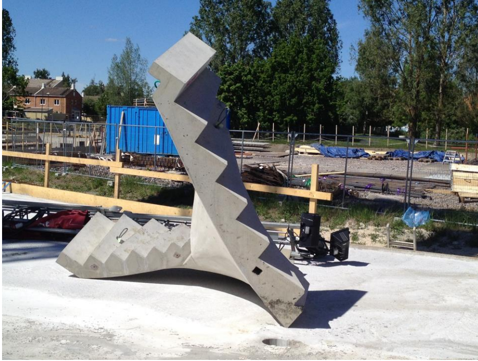
Figure 4.6 unconformity of stairs design to the structural design framework Source: Botrygg, Örebro, Fallskärmen residential project
