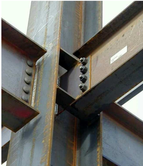
Figure 2.9 Dry connections in steel structures
