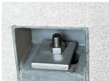
Figure 6.7 Wall shoe mechanical connector.
