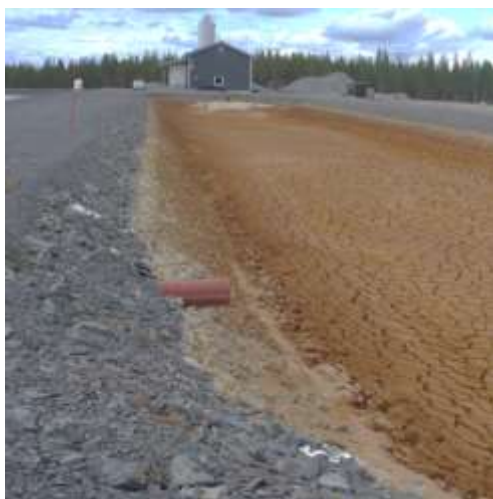
Figure 23 The sediments have been drained and waiting to be excavated.
