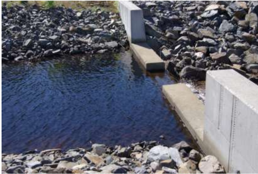
Figure 26 Concrete threshold in a dike connected from a system of reservoirs.
