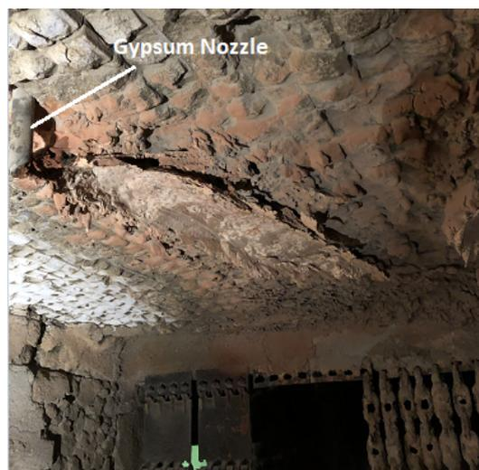
**Figure 2.9:** Picture of nozzle spraying in gypsum in cooler
