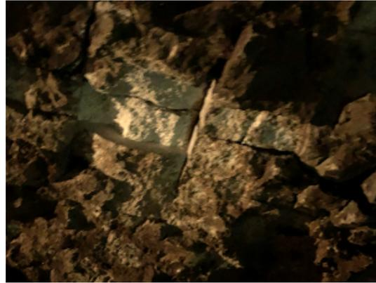
**Figure 2.6:** Picture of how parts of the brick lining is pulled off
