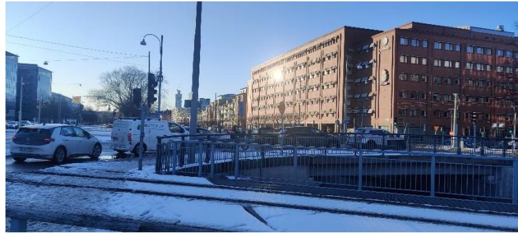
Figure 3.5: Traffic congestion in SBO direction
