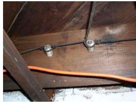
FIGURE 1 CONDUCTOR INSULATED WITH CLOTH.
