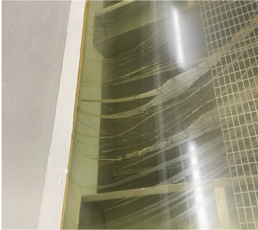
Figure 16. Showing the pollution coating on the surface of sand filter 6, in the plant.
