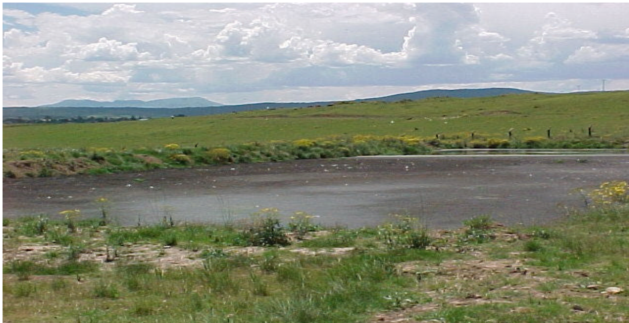
Figure 26 Sludge lagoon at Dimbaza Sewage Treatment Works.
