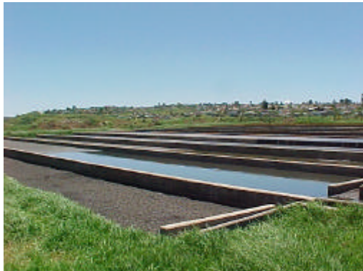
Figure 22 Drying beds at Zwelitsha Sewage Treatment Works.
