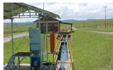
Figure 25 Treatment plant inlet.
