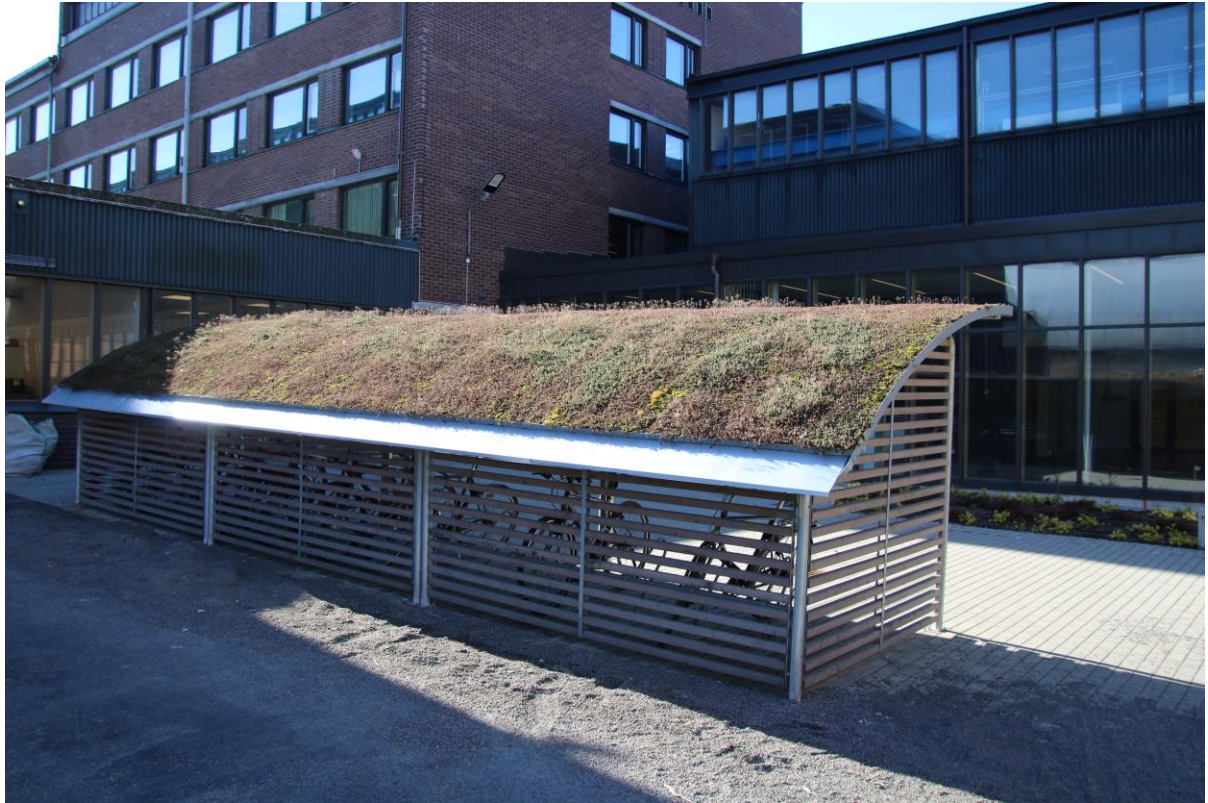
Figure A.2 Bike garage with a green roof on Betonggården at Chalmers University of Technology (Authors' own picture, 2021).
