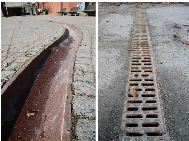
Figure 2.2 Left picture: A canal at Chalmers University of Technology. Right picture: A covered gutter at Chalmers University of Technology (Authors' own picture, 2021).
