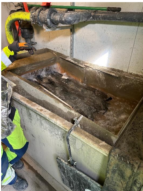
Figure 5. Chitosan is added to incoming excess water in a dosing tank with containers. It is dosed passively as water flows over the containers, washing away the chitosan gel (Photo by A. Nuur).
