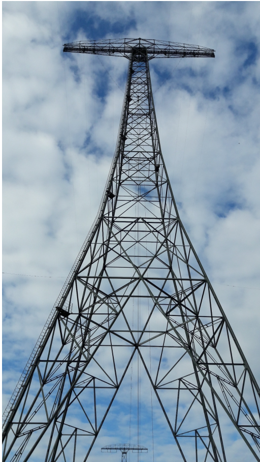
(a) An image of the third antenna tower at Grimeton Radio Station, the one used for the experiment. The tower is 127 meter high and is part of a long wave transmitter antenna.
