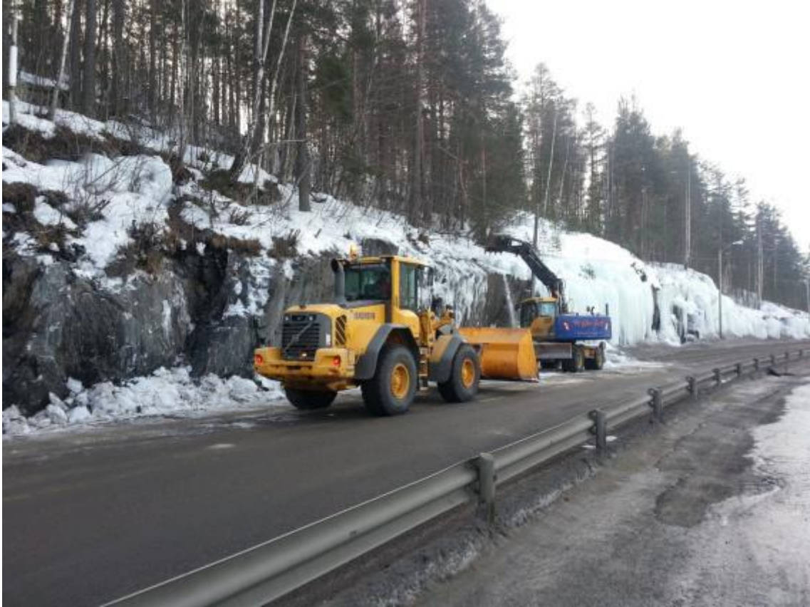
Figure 30: Physical removal of ice in Kongsberg on the 8 th of March 2013.
