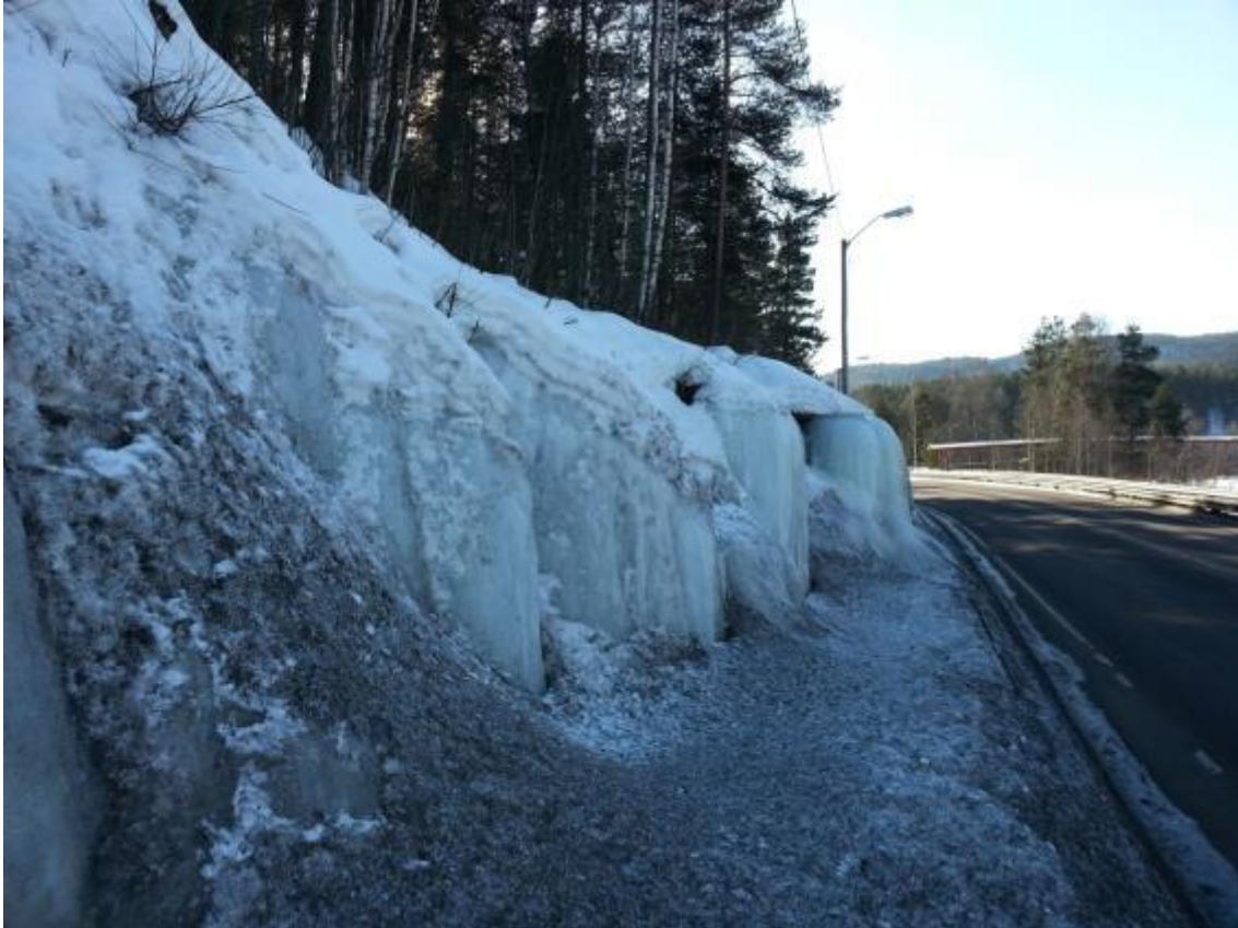
Figure 26: Picture taken in the study area. Here the ice reaches the side of the road, reducing line of sight for bypassing traffic.
