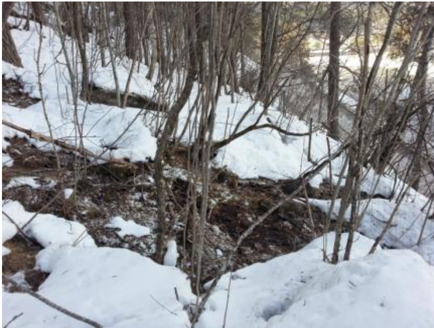
Figure 13: One of the patches above the rock cut which was not covered with snow. There was no sign of running water but the ground was wet and unfrozen. This area will be blasted away during construction of the new road.
