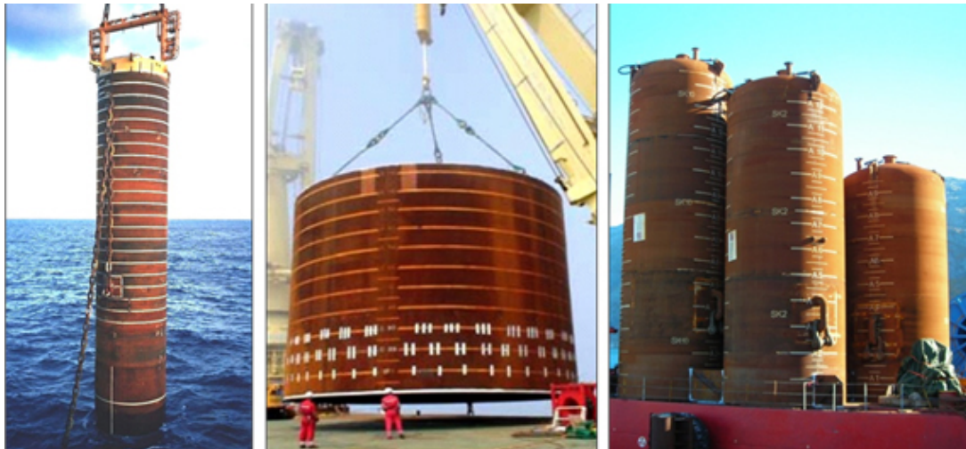
Figure 3 - Suction caisson examples (NGI, 2014)
