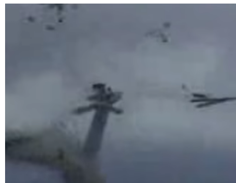
Figure 1.2: Wind Turbine Destroyed [1]
