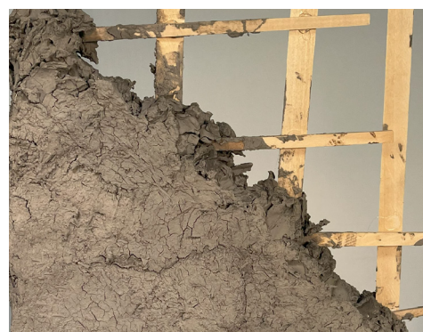
This model shows the construction of the reinforced rammed earth walls. These stand next to each other, providing high performing sound insulation.
