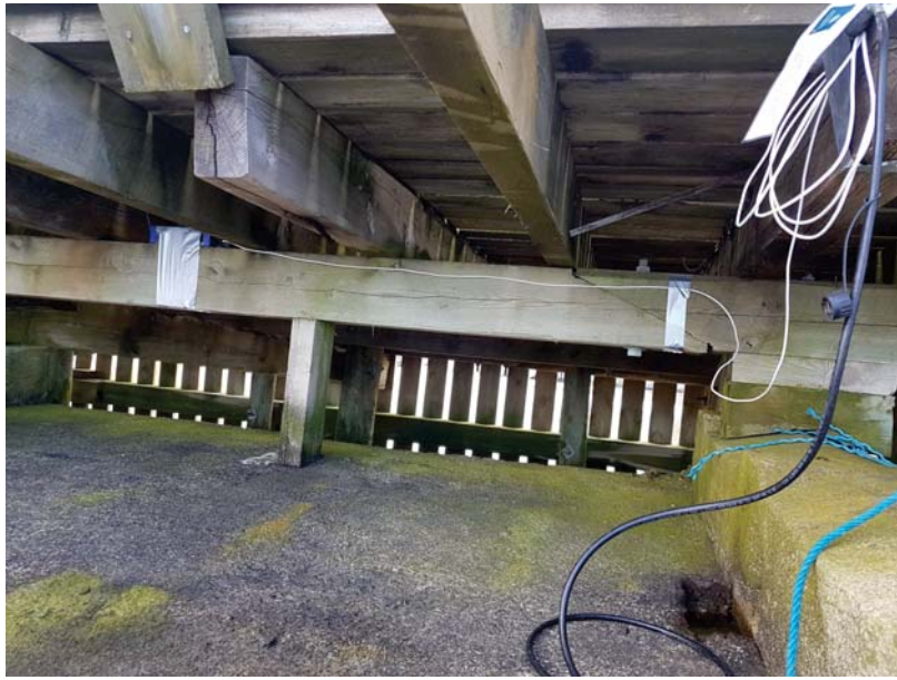
Figure 6.5: The figure presents the device placement at third test location.
