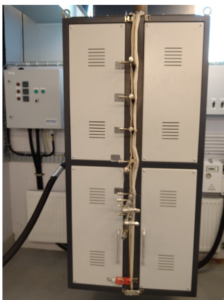
Figure 3.4: Outside of the reactor
