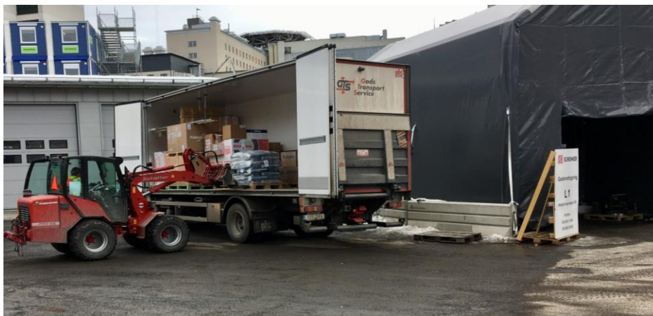
Figure 24: Material is being unloaded at the unloading zone L1.
