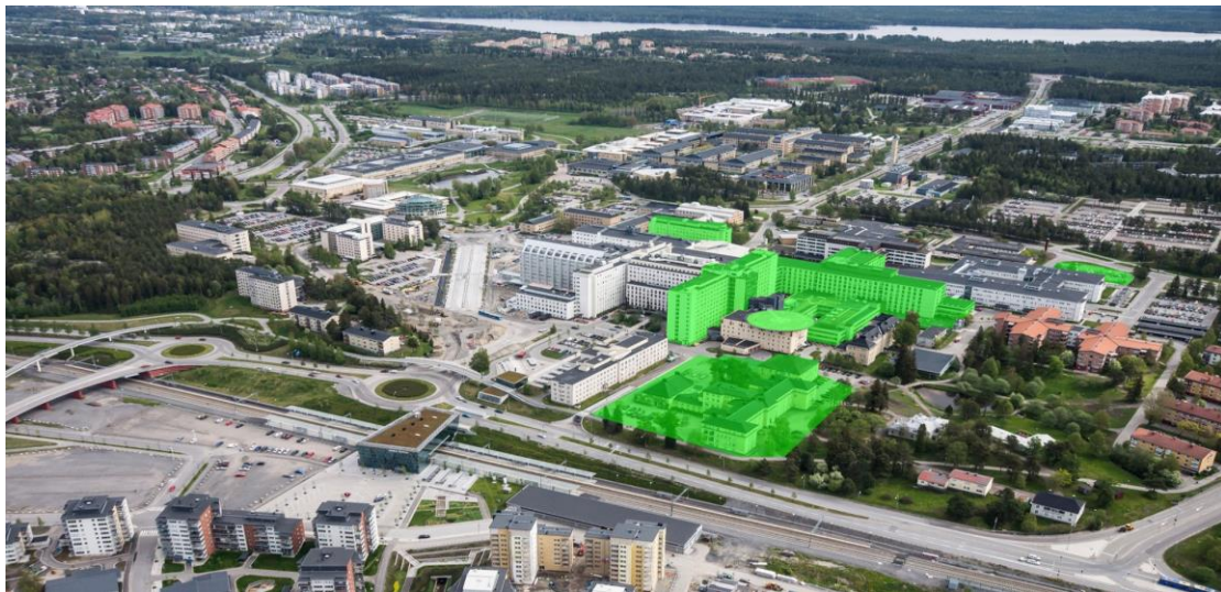
Figure 20: An overview of NUS. Buildings marked in green will be renovated or rebuilt.
