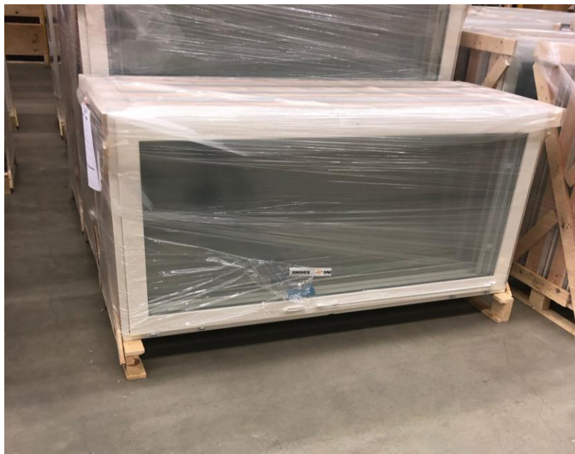
Figure 37: Windows can be delivered on blocks instead of pallets, which increases the risk for transportation damages from forklifts.
