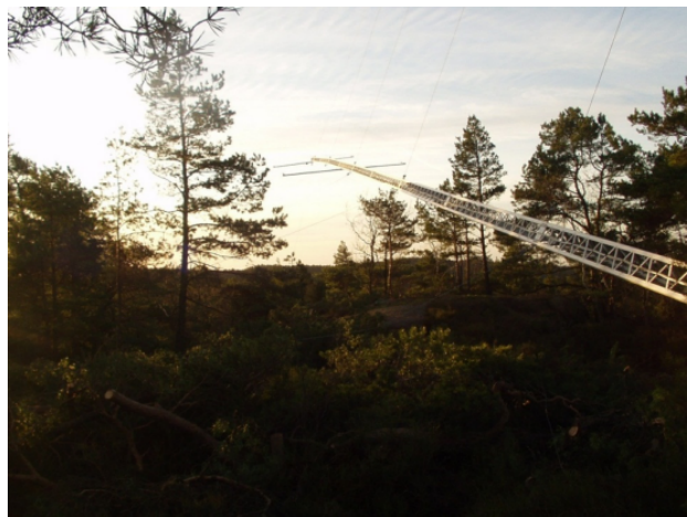
Figure 6.3: Installation of the meteorological mast.
