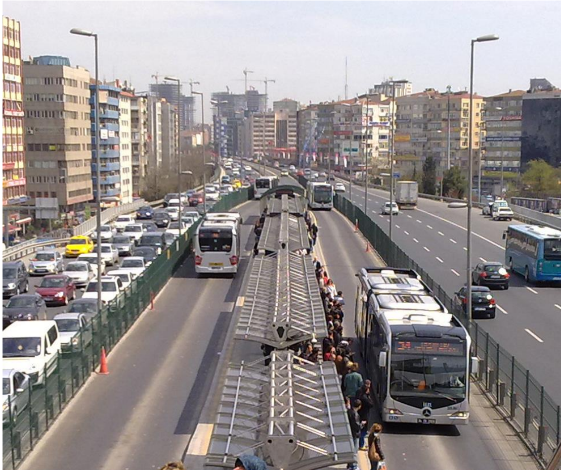
Figure 11. Photo over Mecidiyeköy station. It shows how the busway is located in the middle of the freeway and how the station is placed centered in the busway, with buses driving in opposite direction of regular traffic. (Chumwa, 2012)
