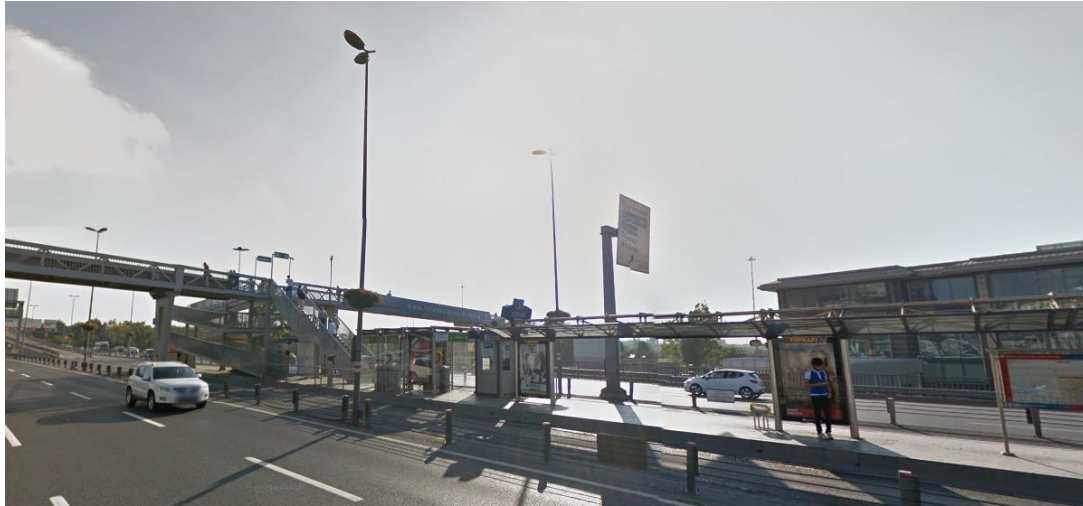
Figure 12. Photo from Google Maps 2015, illustrating a station with overpasses.
