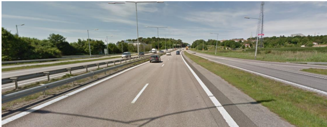
Figure 4: The road E6.20 near Järnbrottsmotet where railings separate the two directions, Google Maps, 2015.
