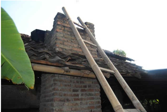
Figure 9: Temperature measurement of exhaust gasses.
