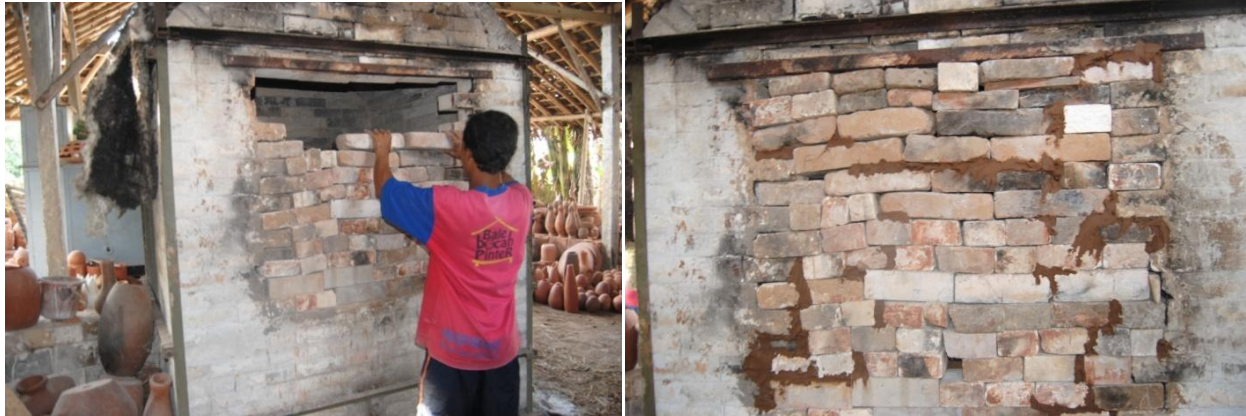
Figure 6: Closing the entrance of the kiln. To the left, the bricks are used and to the right, the small distances are covered by clay soil.
