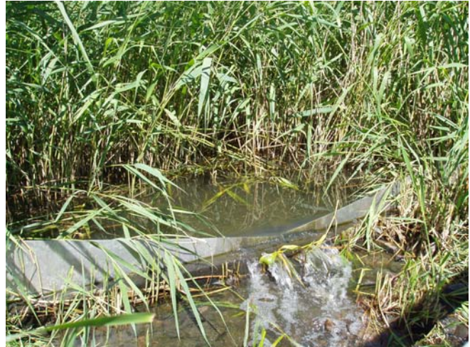
Figure 7. Weir notch (157°) at the outlet.
