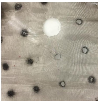
Figure 13. The screen welded on top of the distributor plate in the air reactor after some time running the system. The smaller holes are the ones that had been blasted open by particles that had fallen into the plenum. The big hole is a hole cut out in order to be able to drain the bed.
